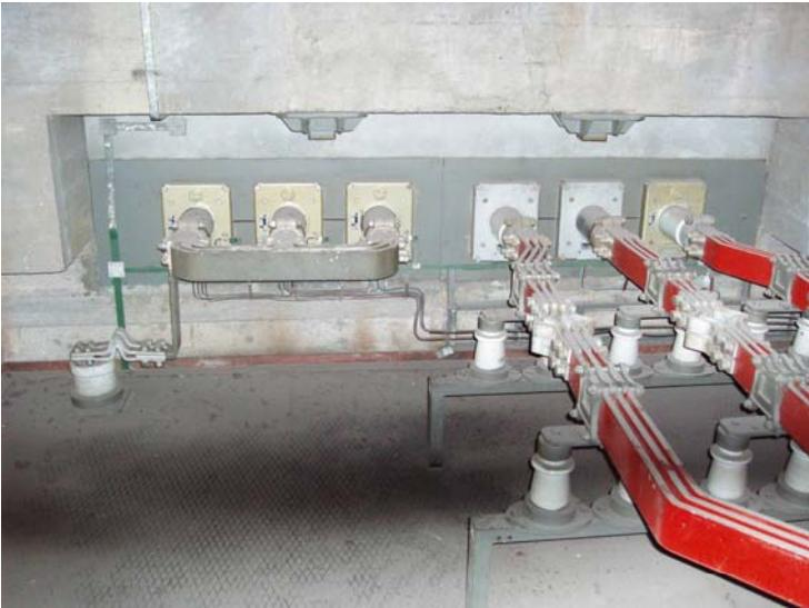
For power outlet from medium sized generator a multiple rigid conductor arrangement can be used (in this case 3 x Al 63x10 per phase)
