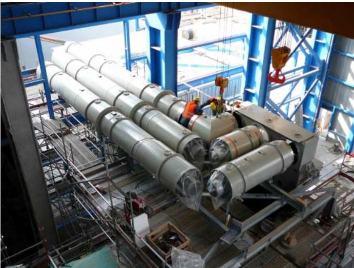
Aluminum enclosed bus ducts are used for the most heavy current demanding installations
