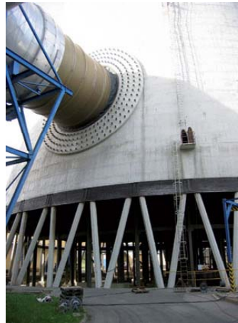
cooling tower with integrated flue gas outlet from FGD
