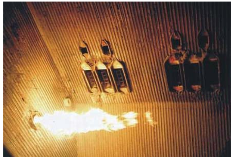
pulverized boiler combustion chamber bottom with LFO burner
